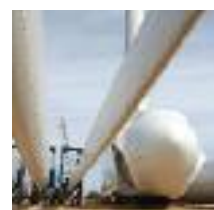
Constructing a wind turbine. © Asterix0597/istock
