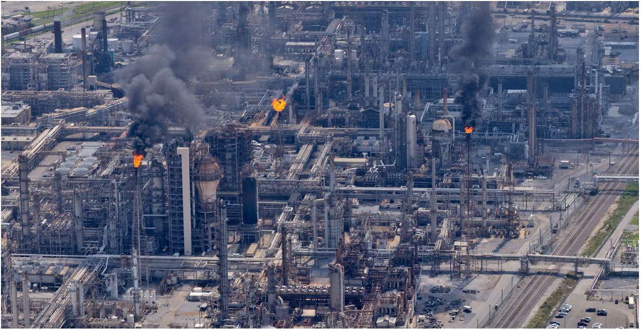
Flaring at a petrochemical facility in Cancer Alley following Hurricane Ida.
