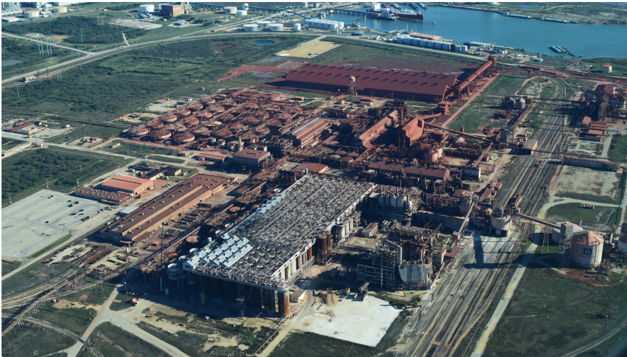
An aerial shot of the Formosa Plastics facility in Point Comfort, Texas.
